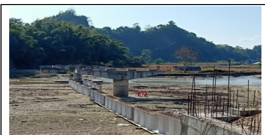
Bridge over Pachin river as on Dec 2019
