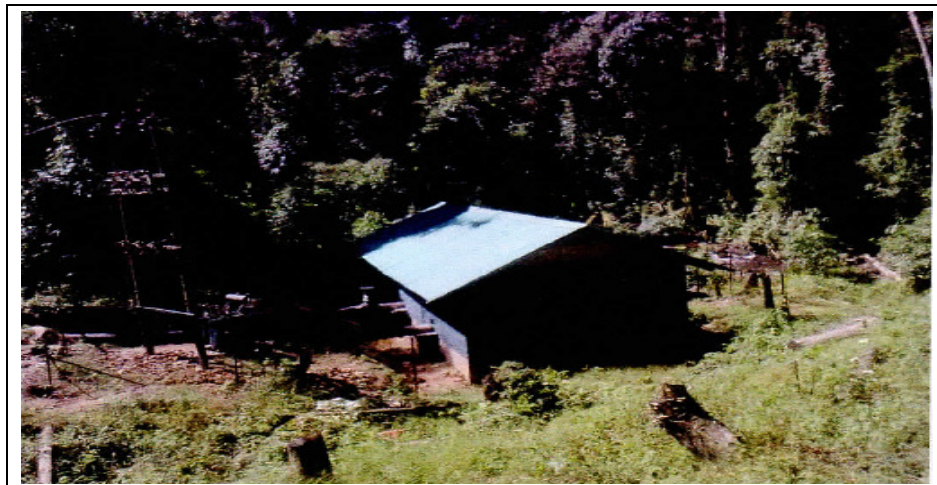
Power House lying idle
